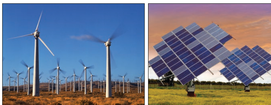
Figure C.2 A wind farm and a solar panel site – the solar panels are mounted on motorised columns to track the Sun across the sky.
